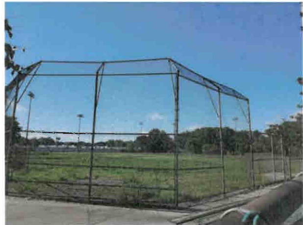
Photograph 4 - View of the baseball field facing southwest from the northeast corner of site. Photo taken by R. Peter Tache, MAI, MRICS, on September 26, 2022.
