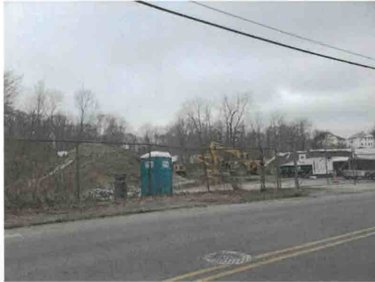
This photograph was taken by R. Peter Tache, MAI, MRICS on March 14, 2022
